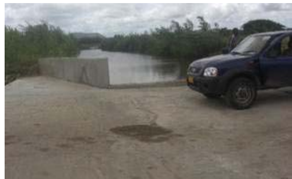
Plate 29: Road crossing dam in Antigua
