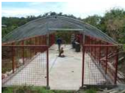
Plate 23. New nursery under construction
